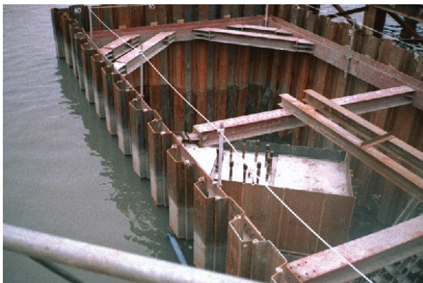
Sheet Pile Interlock
